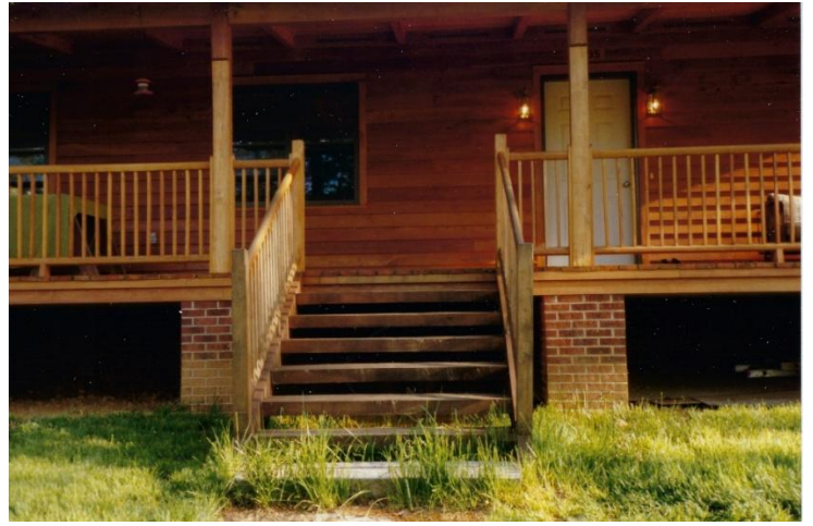
Front Porch Detail, All Wood is Locust Except Porch Flooring
