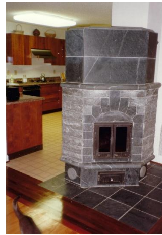
Tulikivi (Finland) Soapstone Fireplace & Four Wood Type Flooring
